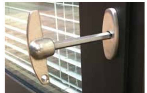
Custodial security lock and optional escutcheon, so key is non-removable in the unlocked position
